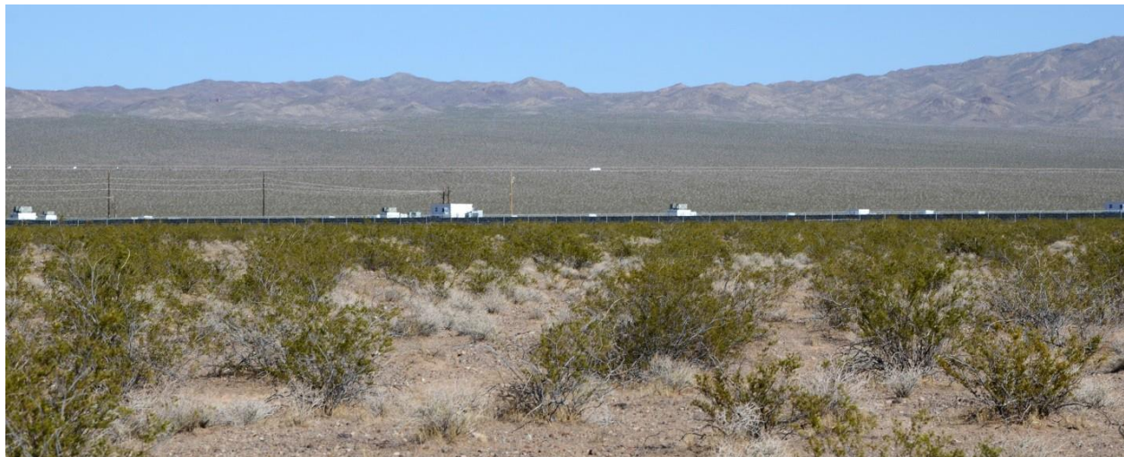
Figure 5.19-5. Ground-Level View of PV Facility Showing Solar Array, Facility Buildings, PCUs, Perimeter Fencing, and Associated Monopole Transmission Towers and Conductors (Credit: Argonne National Laboratory)
