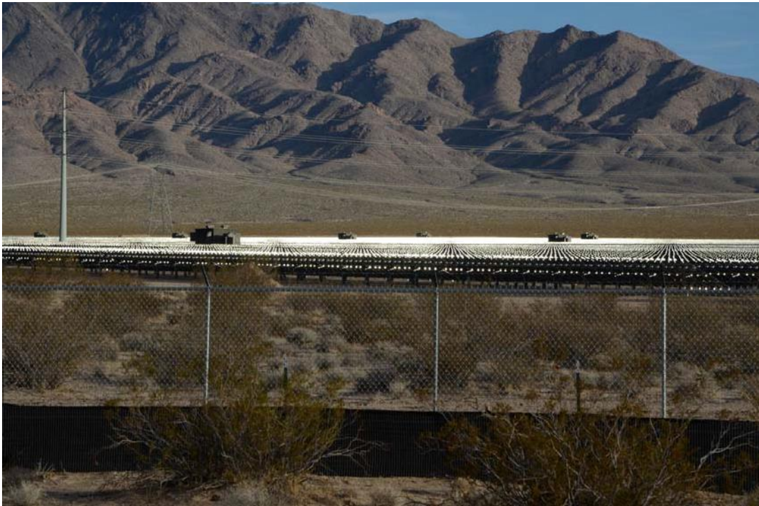
Figure 5.19-8. Geometric Pattern of Reflections from Solar Panel Components at a PV Facility (note that PCUs have been painted to reduce contrast with vegetated mountain backdrop) (Credit: Argonne National Laboratory)
