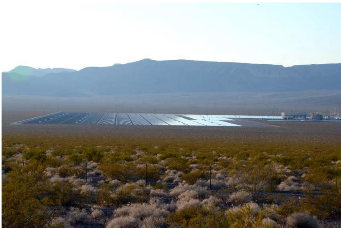
Figure 5.19-7. Color Shift of PV Panel Array from Black (left) through Gray (center) to Bluish White (right), as Seen from a Passing Vehicle (buildings visible at right are not part of the PV facility) (Credit: Argonne National Laboratory)
