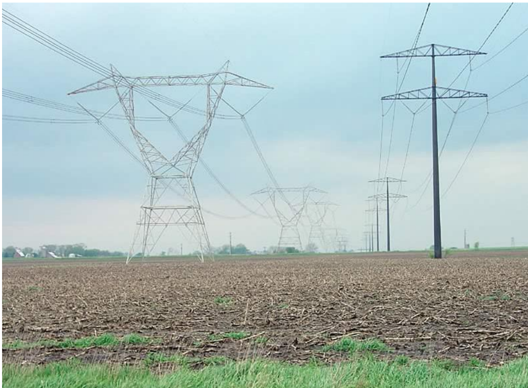
Figure 5.19-10. Lattice (left) and monopole (right) Transmission Towers (Source: Argonne 2007)
