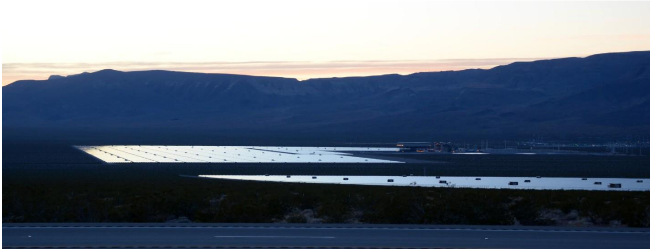
Figure 5.19-6. Low Sun Angle near Sunset Causes Black PV Panels to Appear White and Blue (Credit: Argonne National Laboratory)
