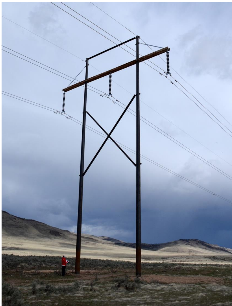
Figure 5.19-11. H-Frame Transmission Tower (Source: Sullivan et al. 2014)
